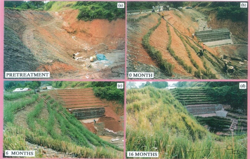
PHOTO 4. QUALITY VGHR PROTECT CULVERT INLET SLOPE C
