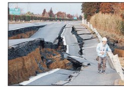
RUINATION: The 8.9-magnitude quake destroyed roads, buildings and other structures, especially in the northeast.
